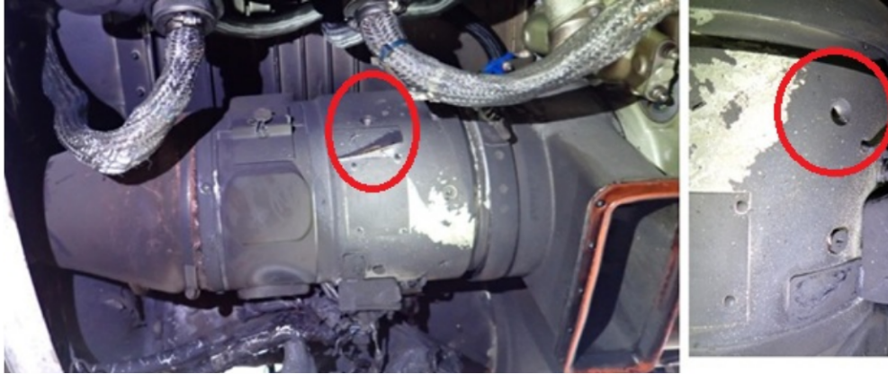
Figure 3. Right engine starter generator and missing screws (red circles)
